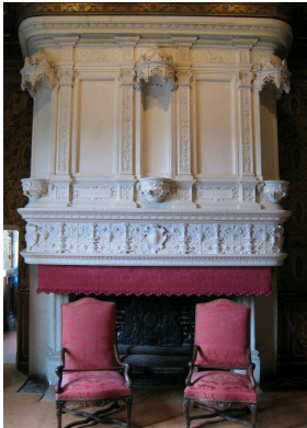
Monumental fireplace made out of Tuffeau decorating the bedroom of François the 1st in the castle of Chenonceau.
