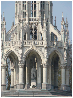
Monument of Leopold the 1st in Brussels, in Belgium, made out of Tuffeau.
