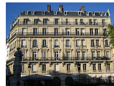
Haussmann building façade,
