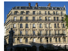
Haussmann building façade,
